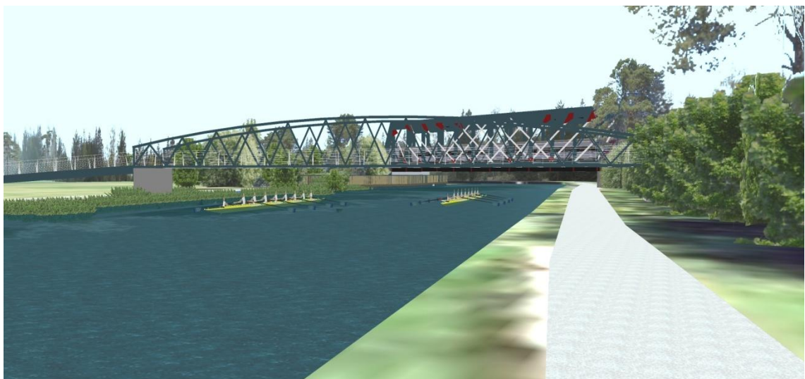
Figure 4 Computer illustration of the proposed foot/cycle bridge main span in truss form with the existing railway bridge in the background
