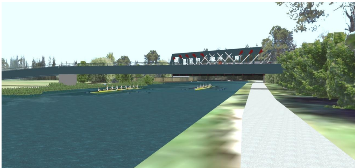
Figure 6 Computer illustration of the proposed foot/cycle bridge main span in half-through girder form with the existing railway bridge in the background
